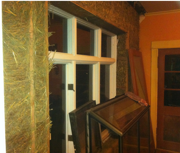
Straw insulated interior wall
